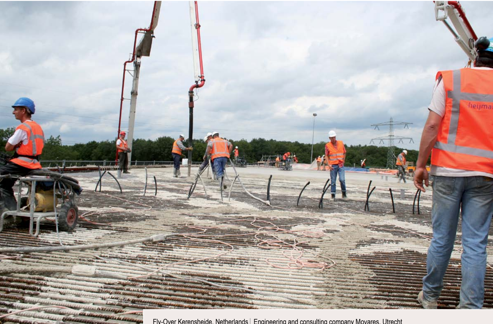
Fly-Over Kerensheide, Netherlands | Engineering and consulting company Movares, Utrecht
